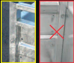
100% welded and hot dipped galvanised to 70 microns thick, (compared to 7 microns thick for pre-galvanised sheets.) No rivets or bolts to cause vibration or wear by rubbing.
