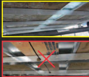
Made of structural angle iron which has a greater resistance to heavy loads than bent steel sheet metal platforms.
